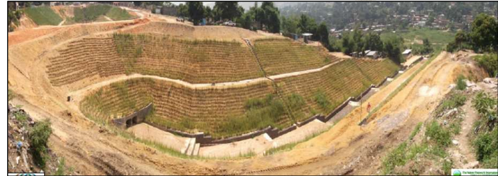
Vegetated Side Slopes of Concrete Drainage Channel
